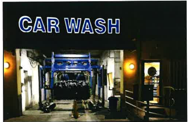
Photo 2. Prestige Car Wash Exit Portal
