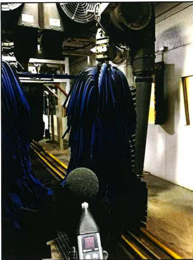
Photo 3. Dryer Blowers Without Silencers
