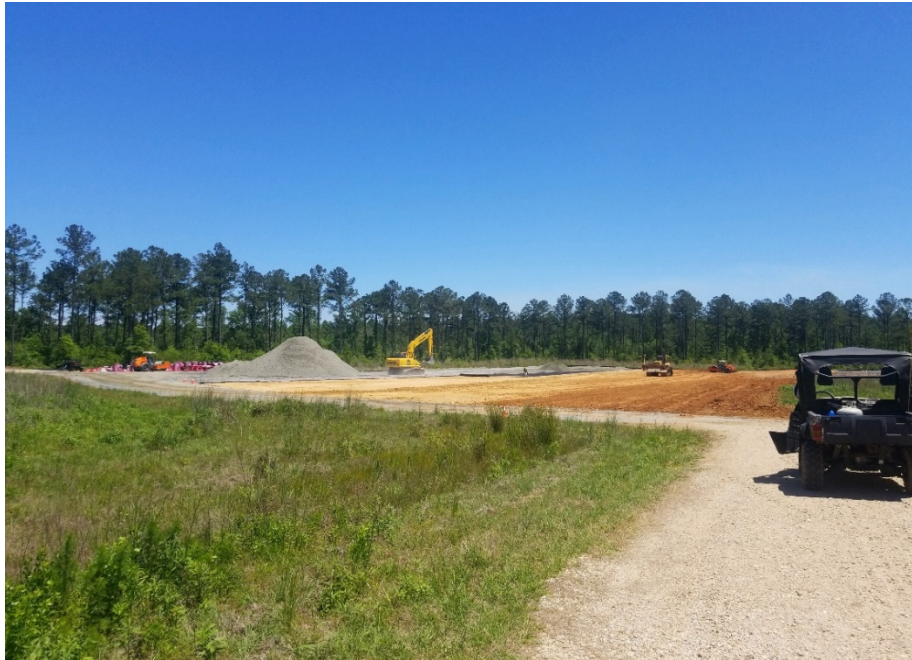
Albany Compressor Station: (facing Southeast)
