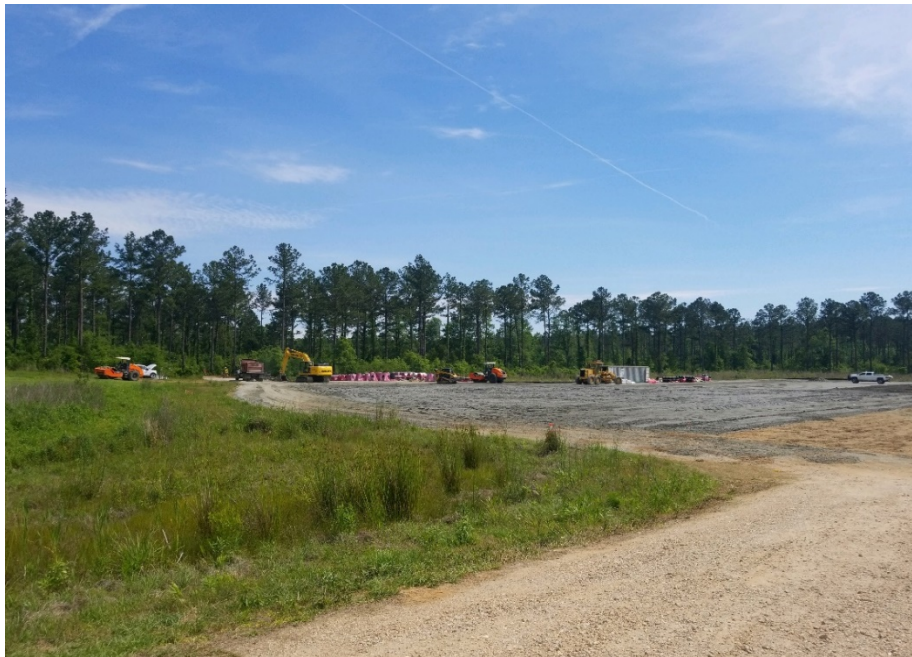
Albany Compressor Station: (facing Southeast)
