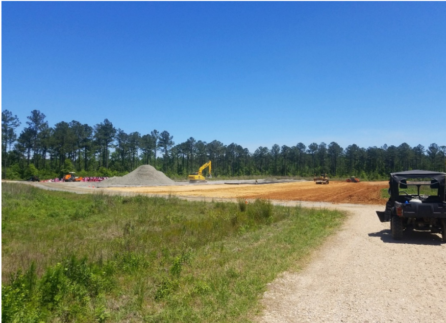
Albany Compressor Station: (facing Southeast)
