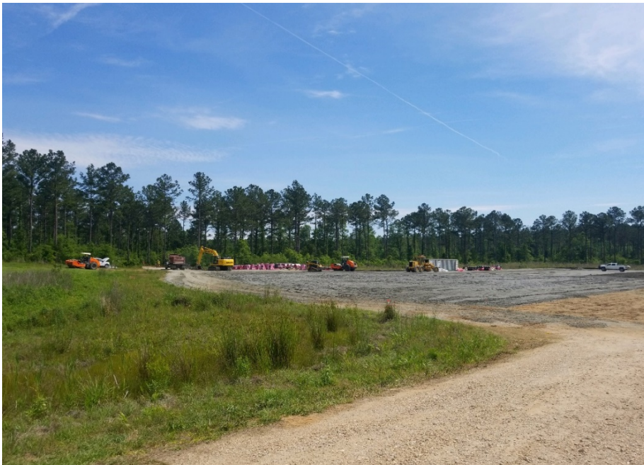
Albany Compressor Station: (facing Southeast)
